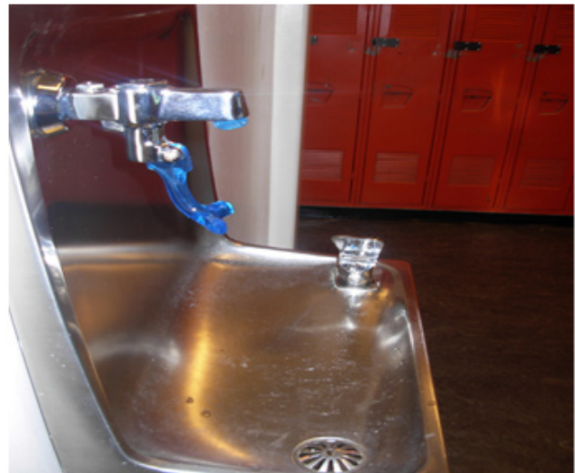
Example of a water fountain at UW that has been upgraded to include a spigot for use with reusable bottles. Photo courtesy of David Jacks.
